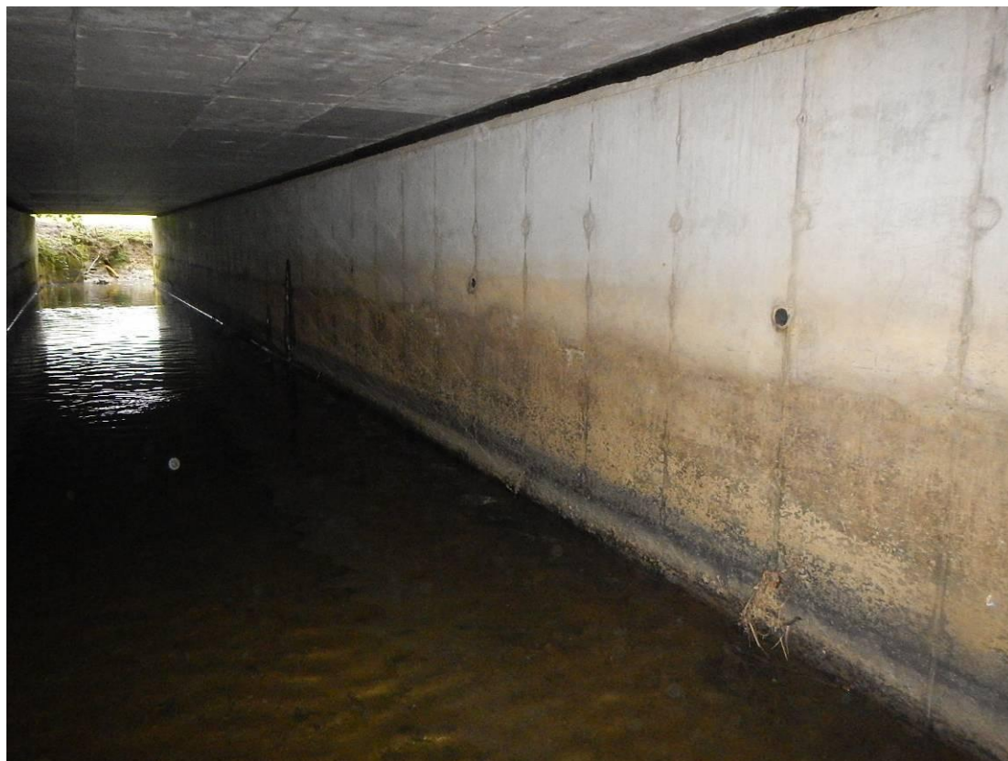
Photo 64 – Structure 4: Concrete Abutment
