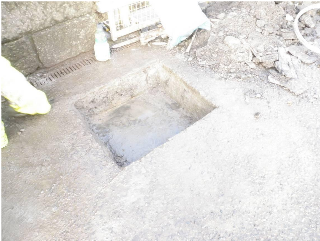
Photo 28 – Structure 2: Structural Investigation
