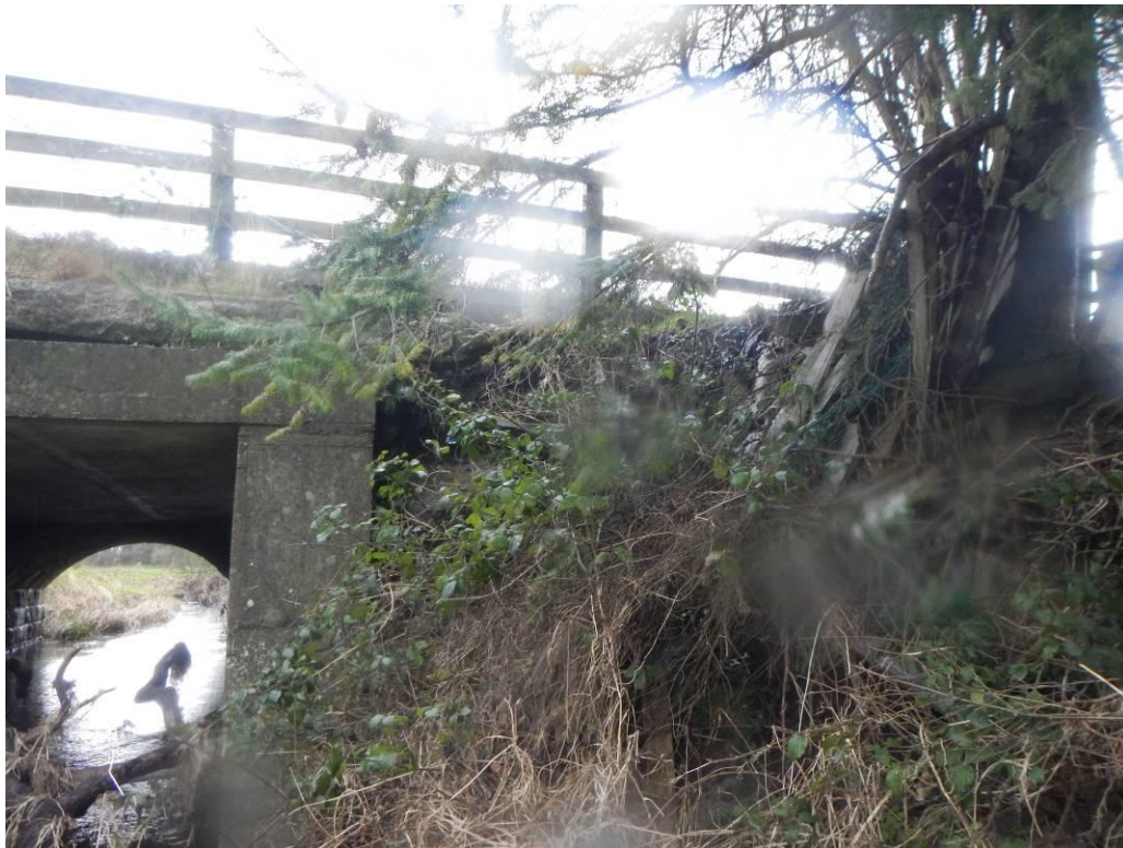
Photo 8 – Structure 1: Erosion of Southwest Embankment
