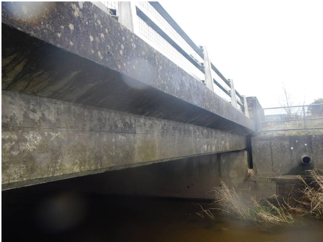
Photo 24 – Structure 2: Precast Edge Panels on South Face
