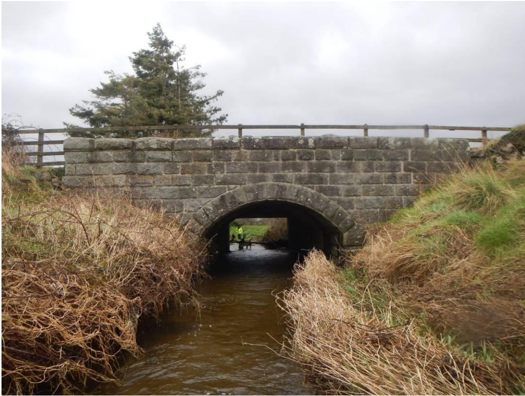
Photo 15 – Structure 1: West Elevation
