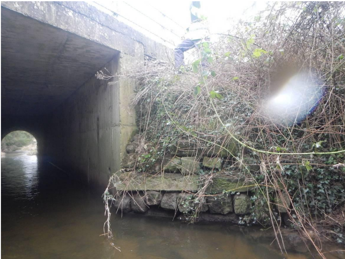
Photo 38 – Structure 3: Southwest Masonry River Training Wall
