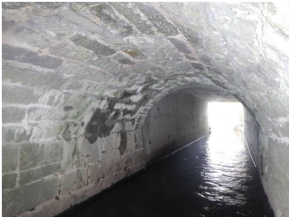
Photo 39 – Structure 3: View on Arch Barrel
