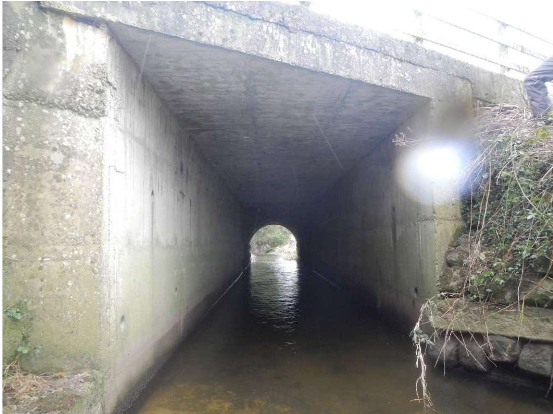
Photo 45 – Structure 3: West Elevation
