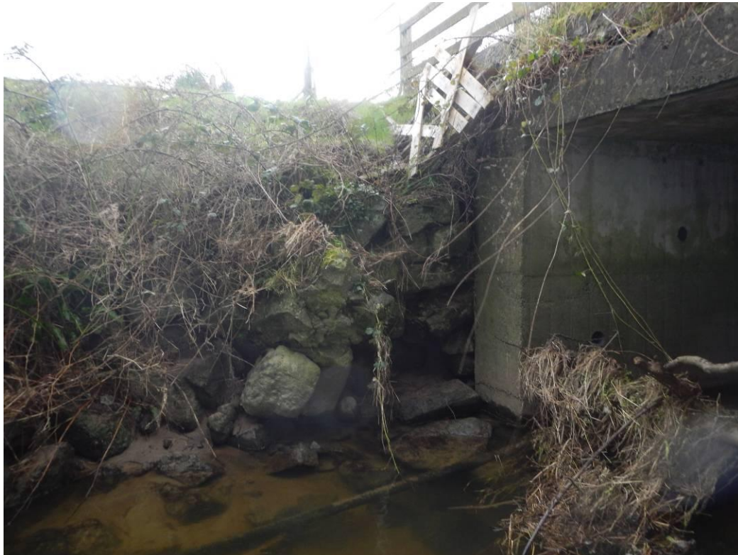
Photo 6 – Structure 1: Erosion of Southeast Embankment
