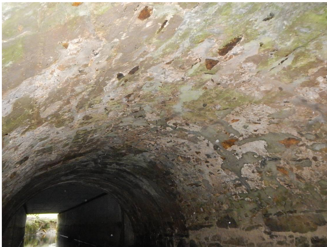
Photo 55 – Structure 4: View on Arch Barrel
