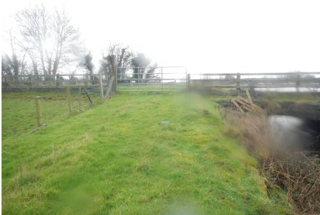
Photo 16 – Structure 1: View of Field Access on Southeast Departure
