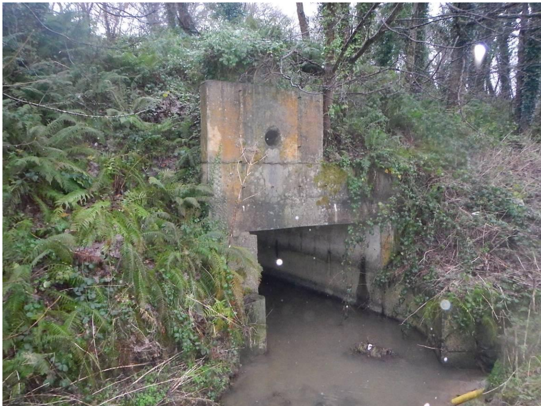
Photo 48 – Structure 4: View on Eastern Inlet
