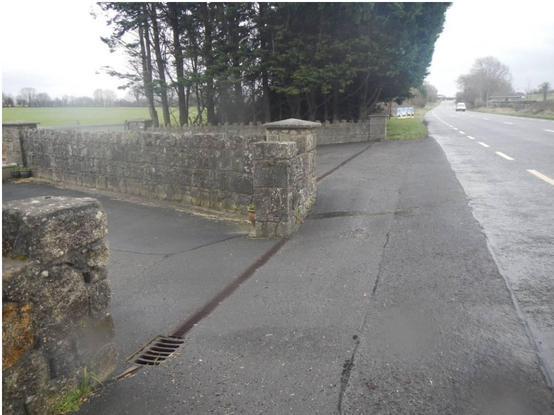
Photo 30 – Structure 2: Private Entrance at Northeast Corner
