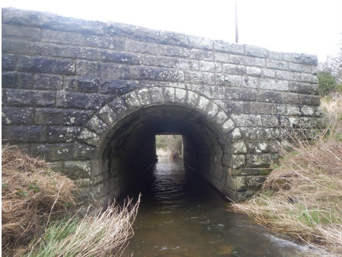
Photo 36 – Structure 3: East Elevation
