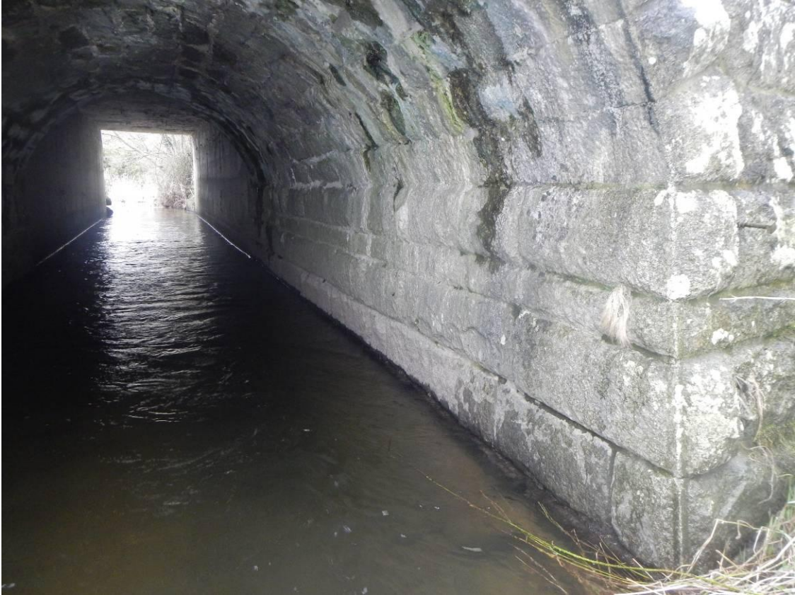
Photo 41 – Structure 3: Northern Masonry Abutment
