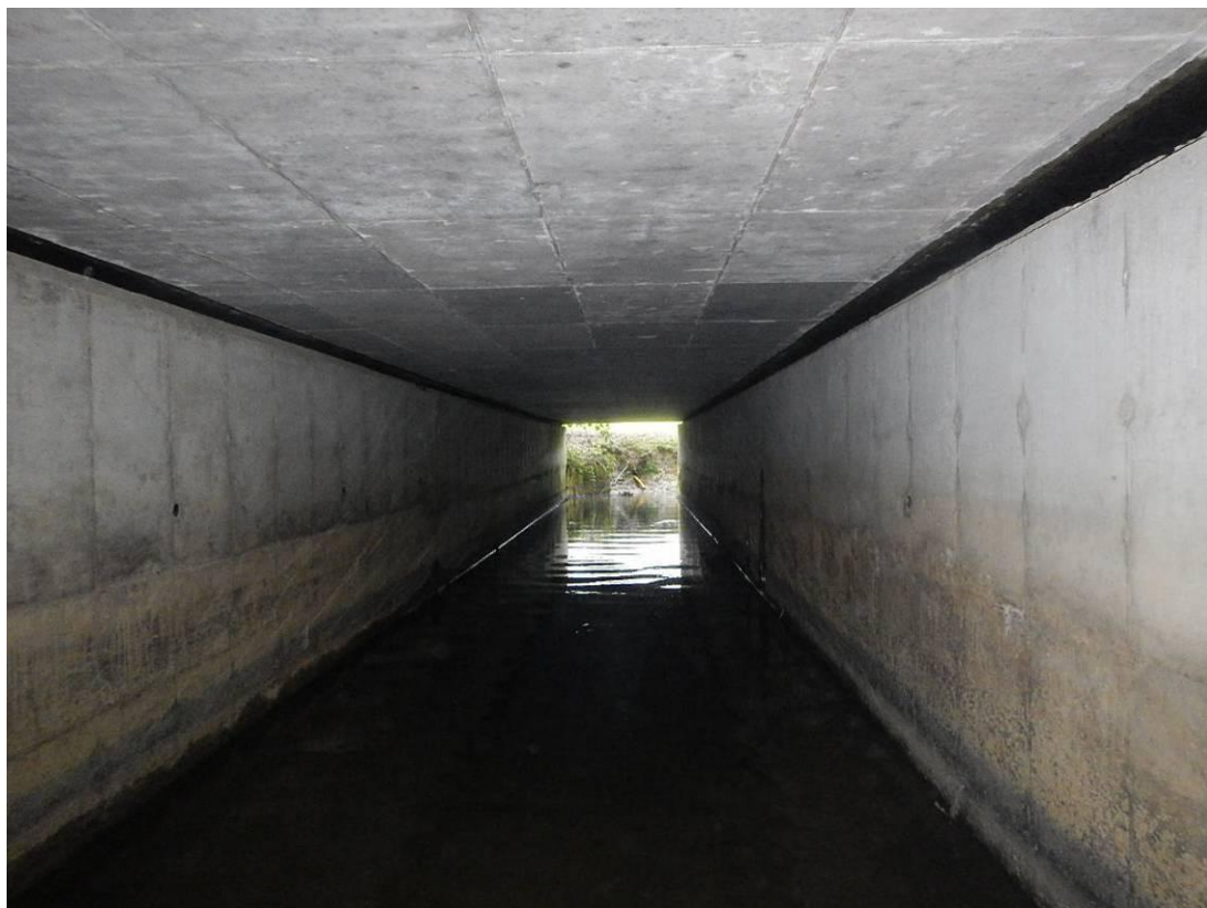
Photo 60 – Structure 4: Reinforced Concrete Deck
