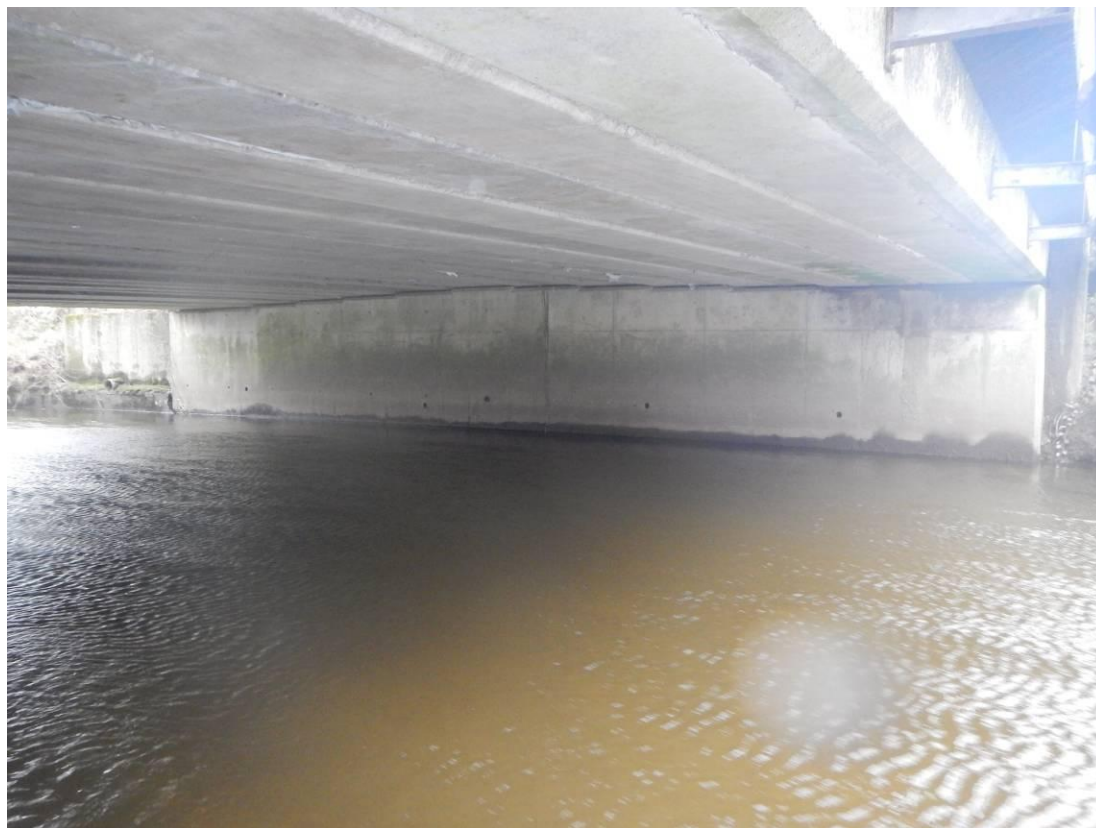
Photo 25 – Structure 2: View on West Abutment
