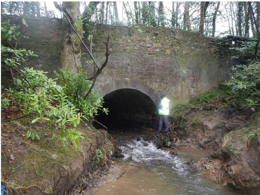
Photo 50 – Structure 4: West Elevation
