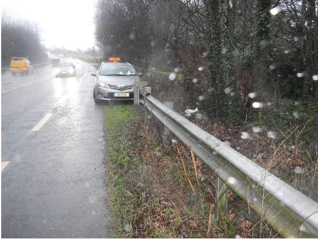
Photo 47 – Structure 4: P4 Terminal on Western Approach
