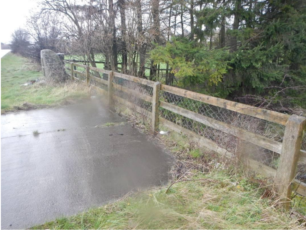
Photo 3 – Structure 1: View of East Parapet
