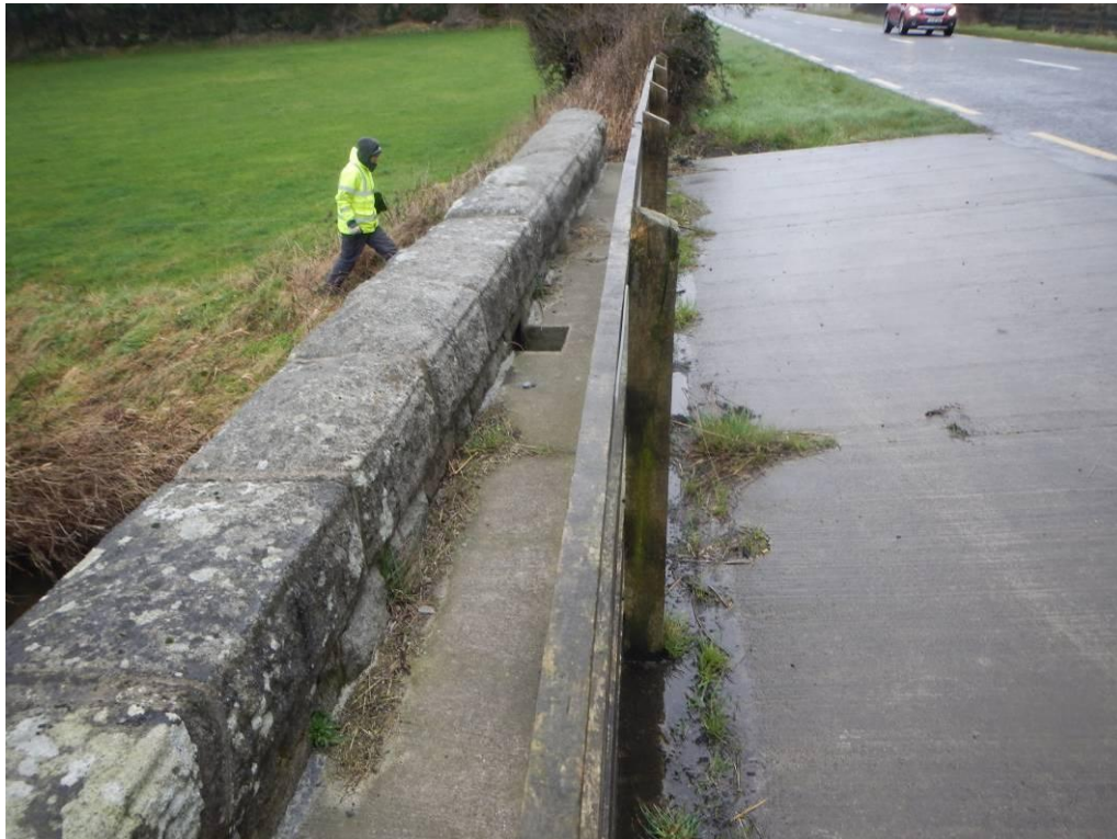
Photo 2 – Structure 1: View of West Parapet
