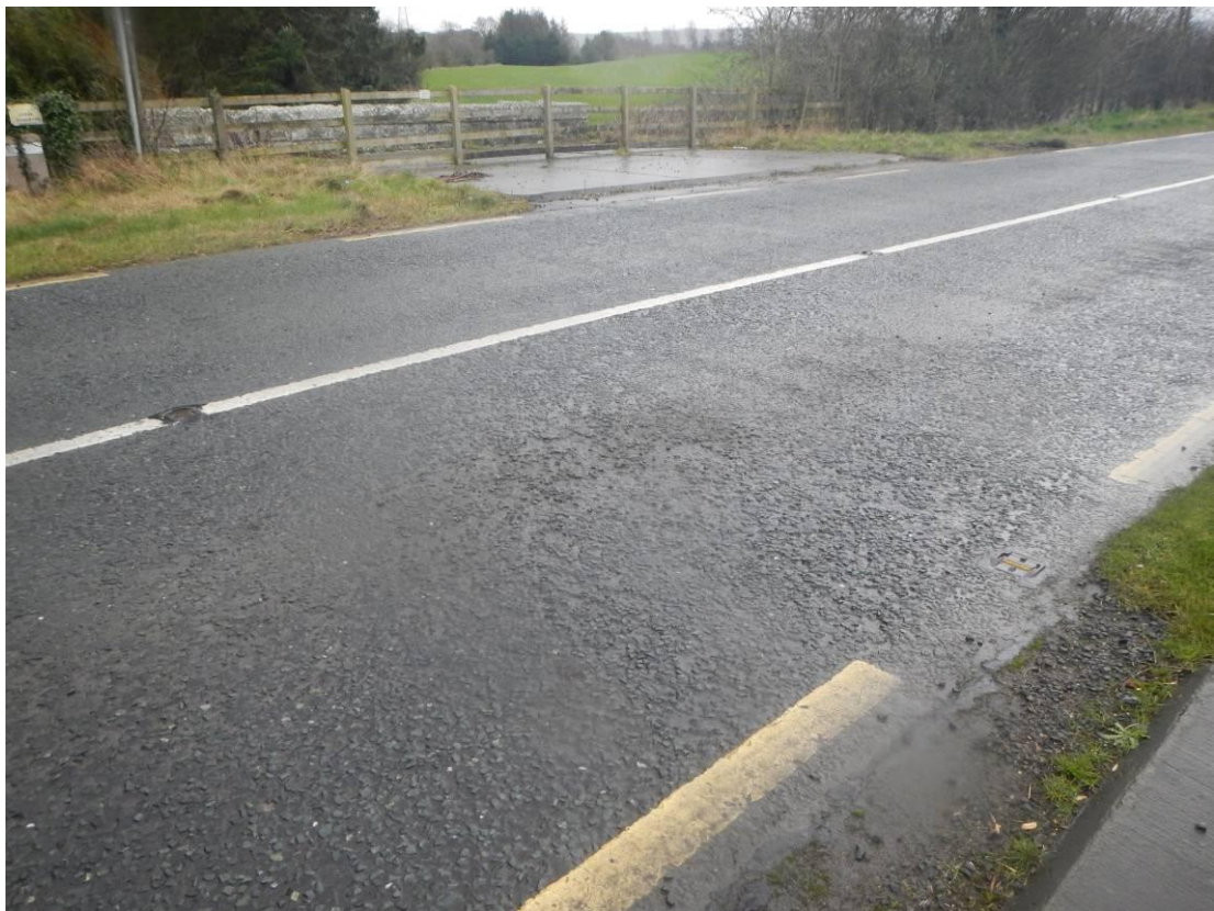
Photo 32 – Structure 3: View of Carriageway Surfacing
