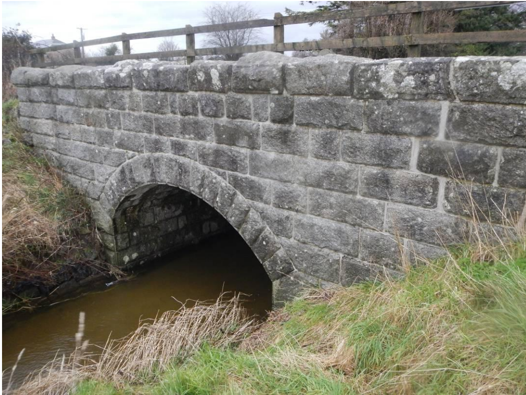
Photo 5 - Structure 1: Spandrel Wall
