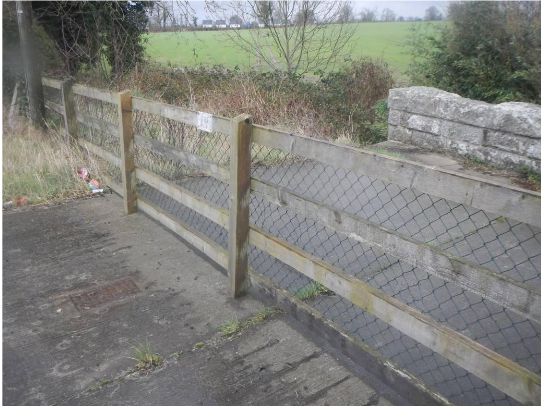
Photo 35 – Structure 3: Eir/Scour Valve on East Raised Verge
