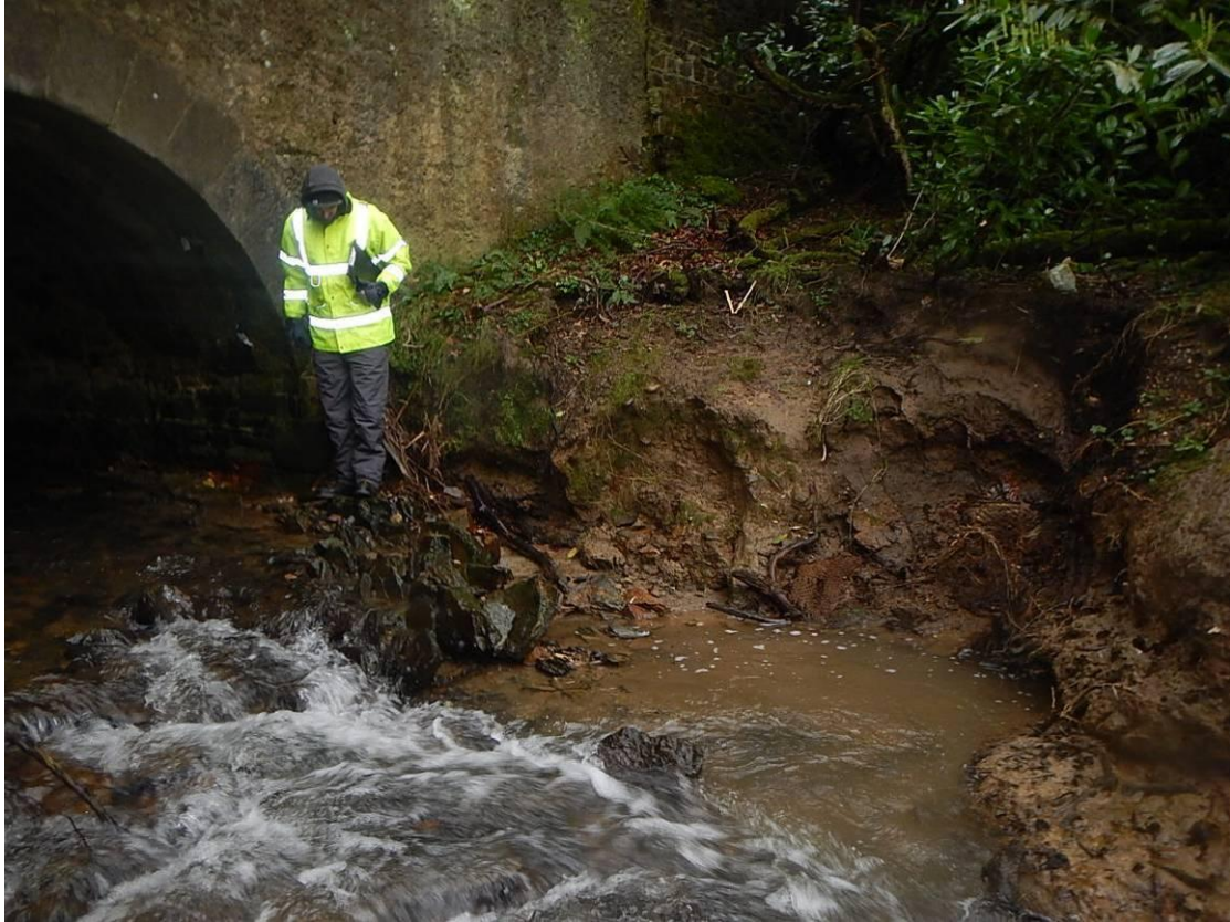
Photo 51 – Structure 4: Erosion of Southwest Embankment
