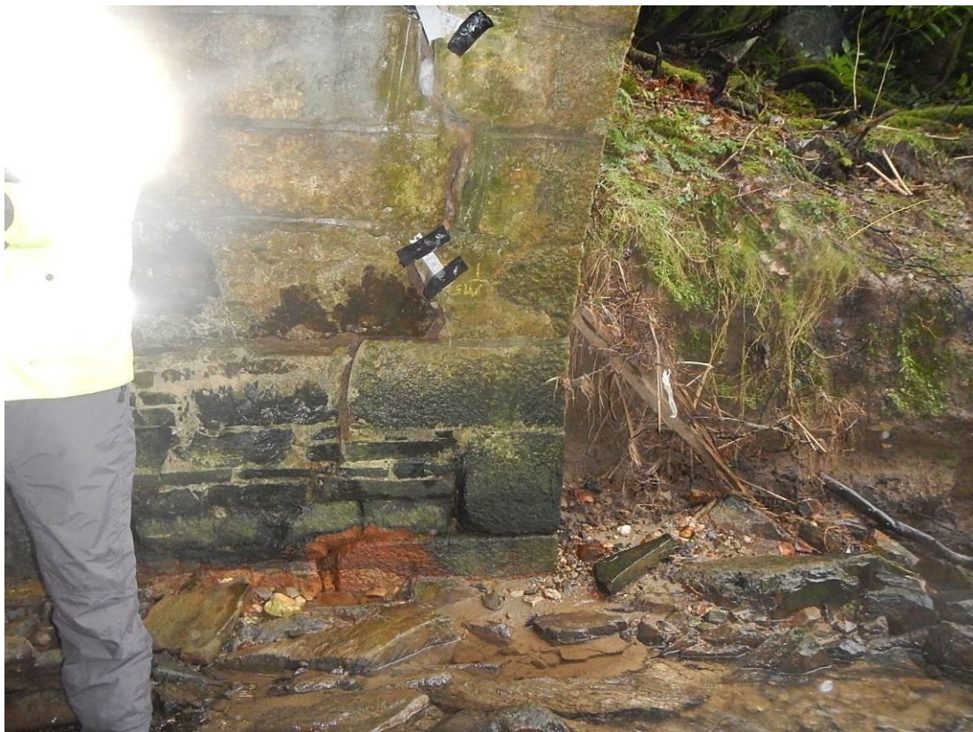
Photo 63 – Structure 4: Circumferential Cracking to the Arch
