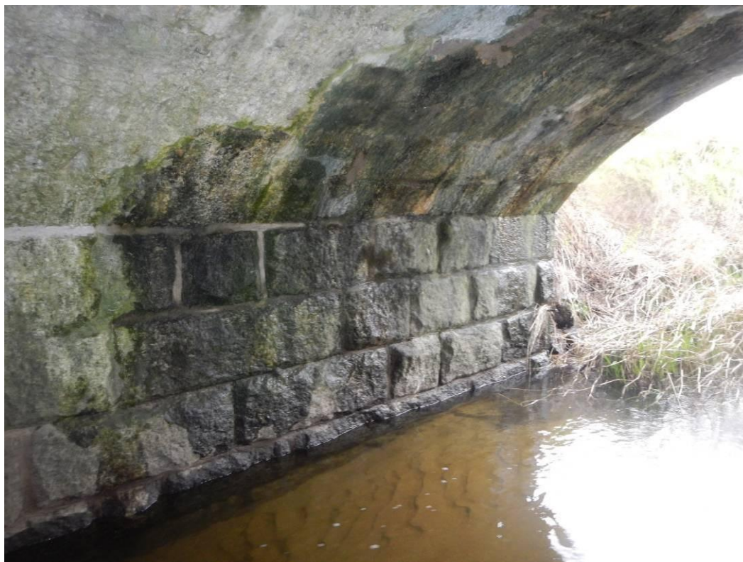
Photo 11 – Structure 1: Leakage at West End of South Masonry Abutment
