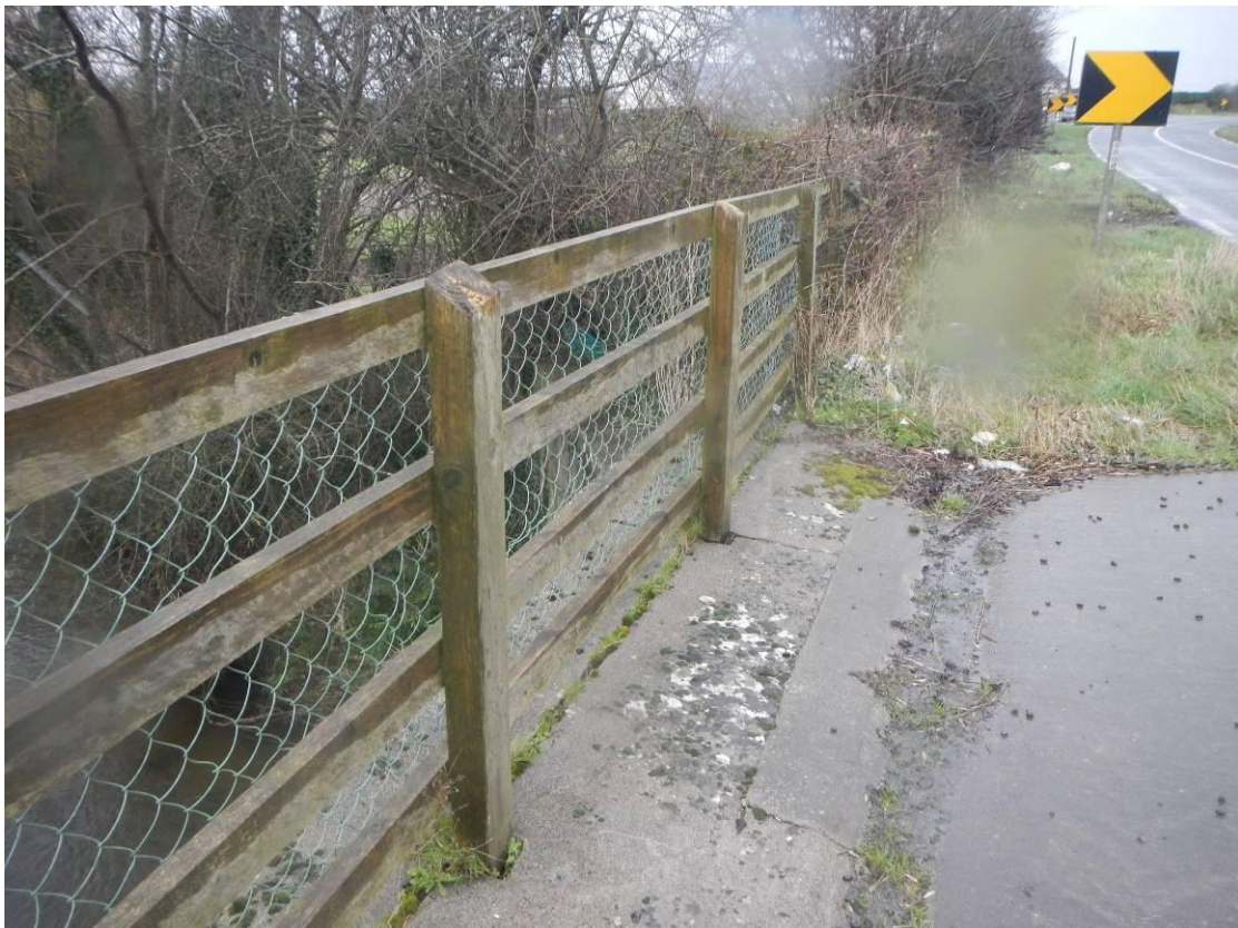
Photo 34 – Structure 3: Timber Fence on West Raised Verge
