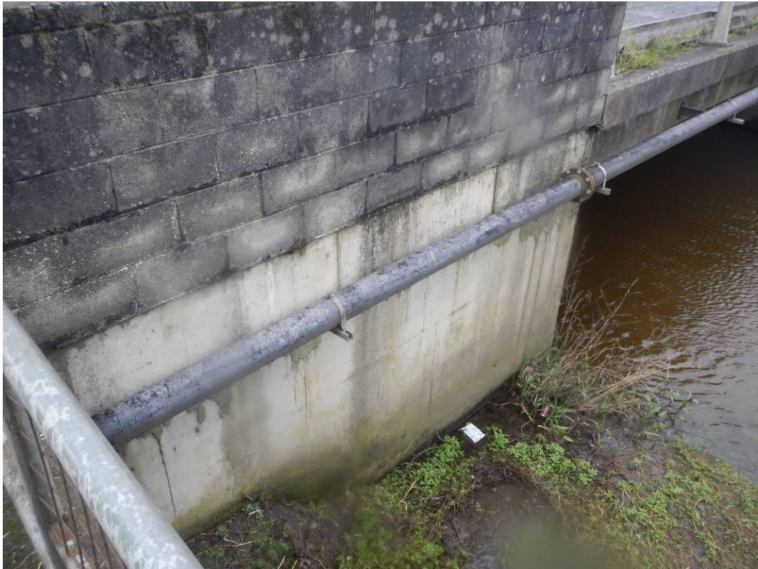
Photo 21 – Structure 2: Concrete Wingwall at Northeast Corner
