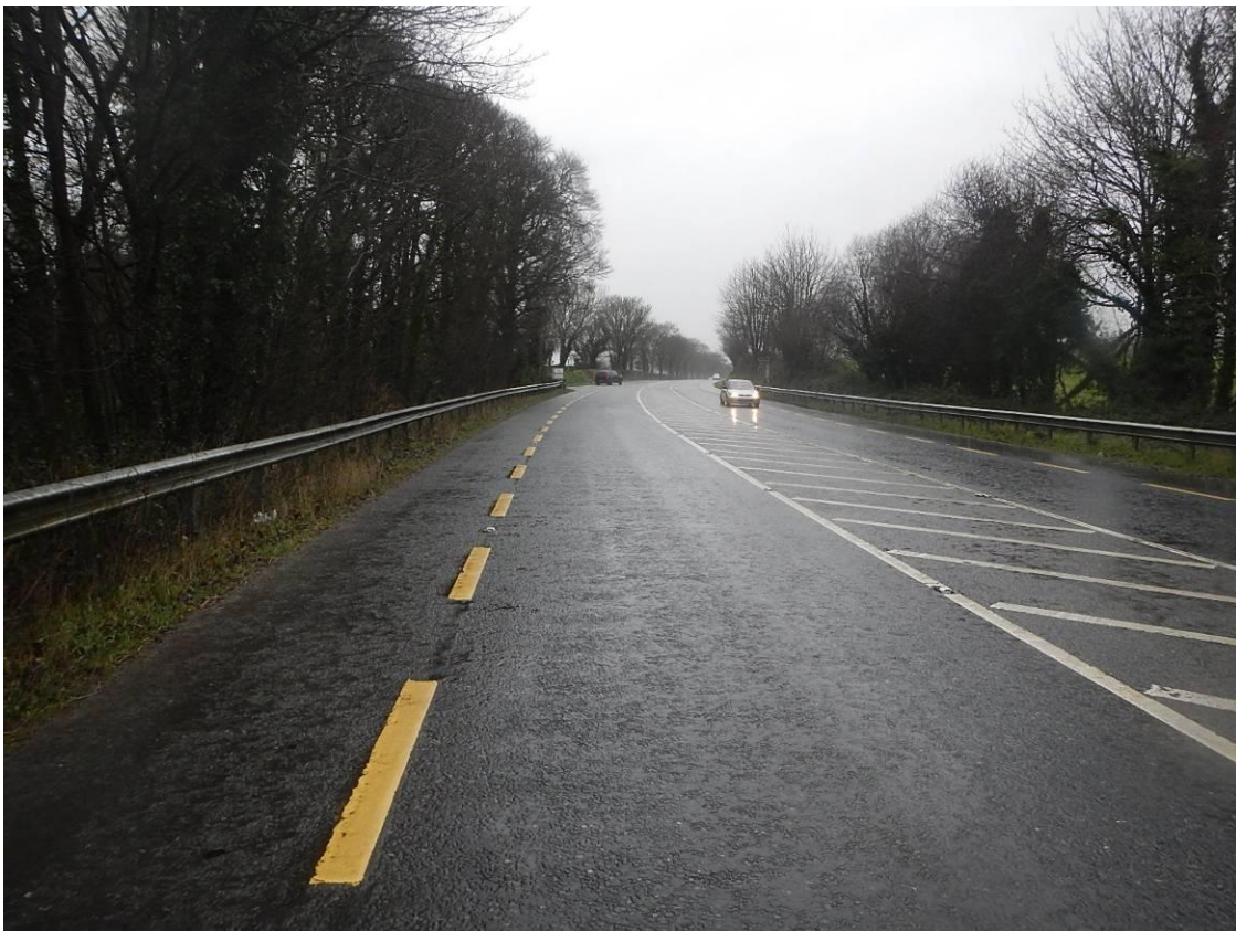
Photo 46 – Structure 4: View on Carriageway Surfacing
