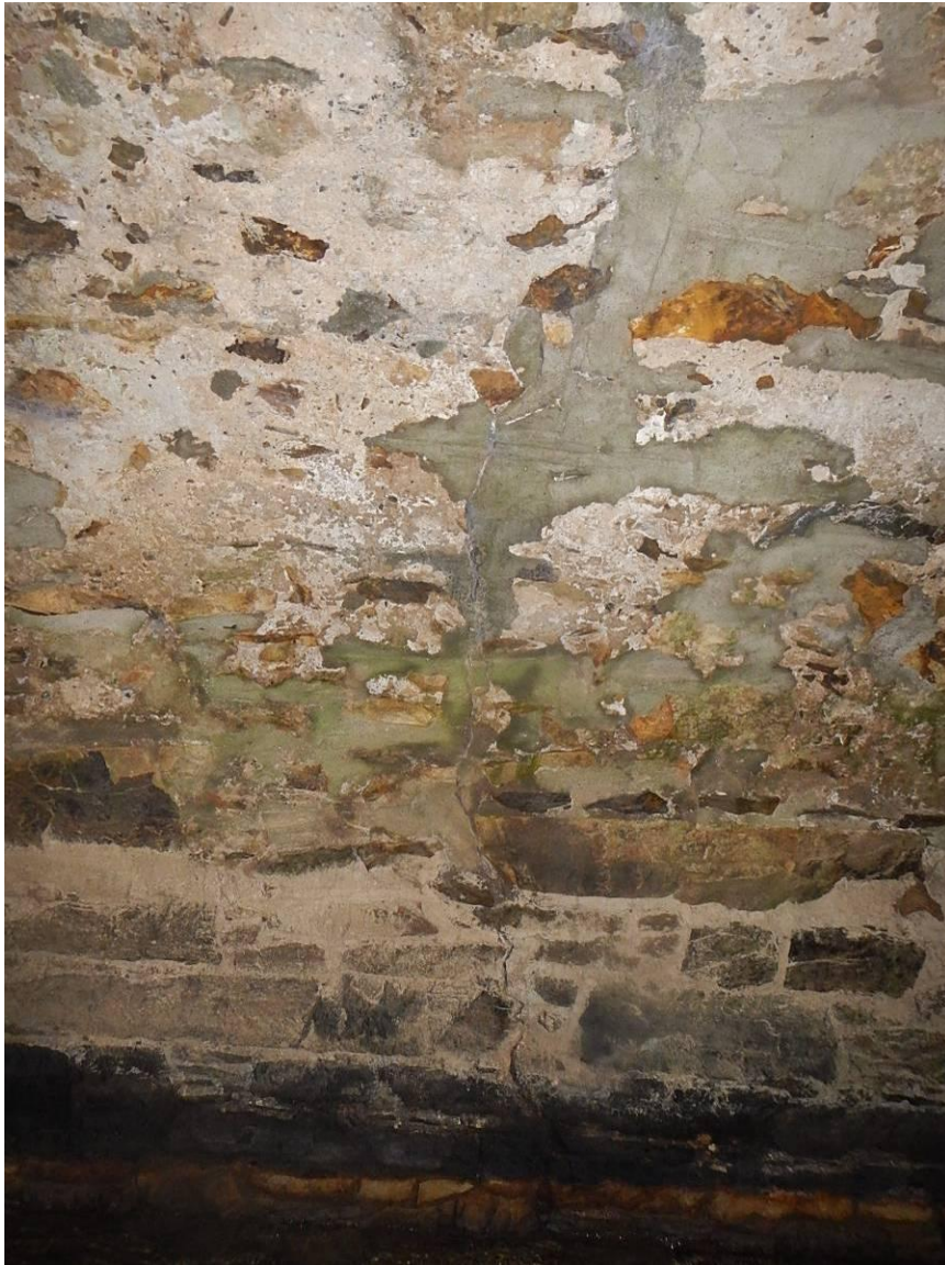
Photo 58 – Structure 4: Second Full Length Circumferential Crack
