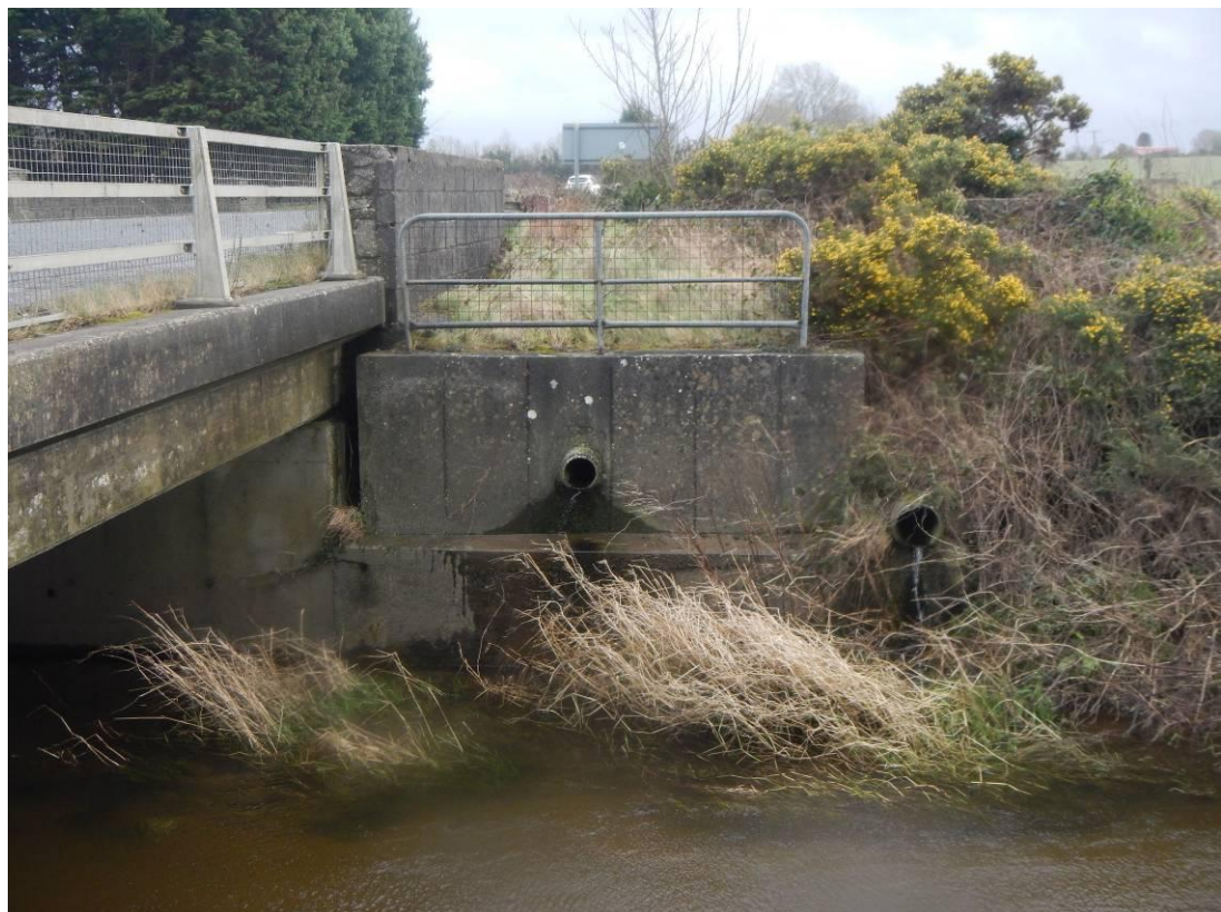
Photo 22 – Structure 2: Concrete Wingwall at Southeast Corner
