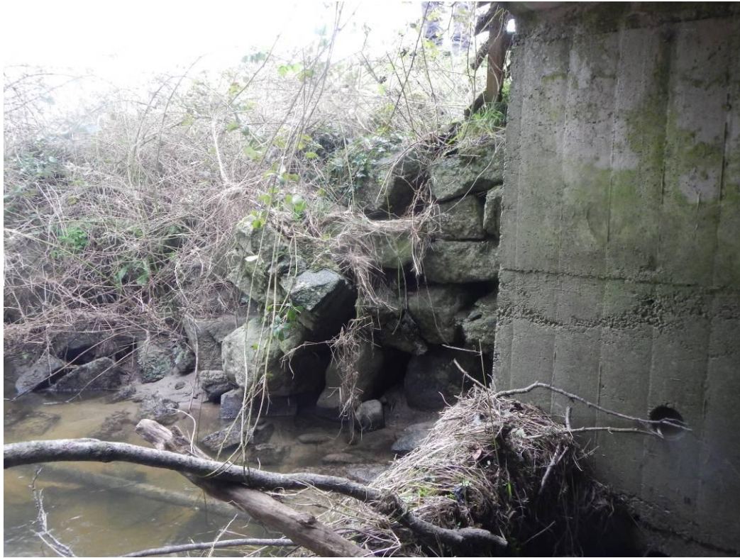
Photo 7 – Structure 1: Erosion of Southeast Embankment
