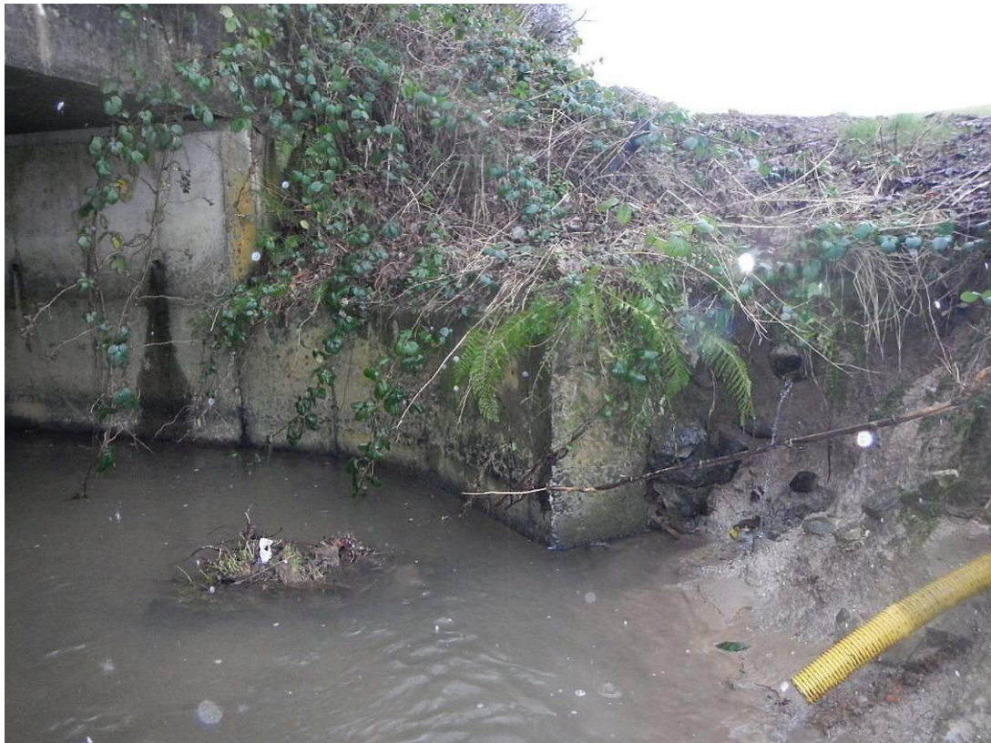
Photo 54 – Structure 4: Northeast Embankment
