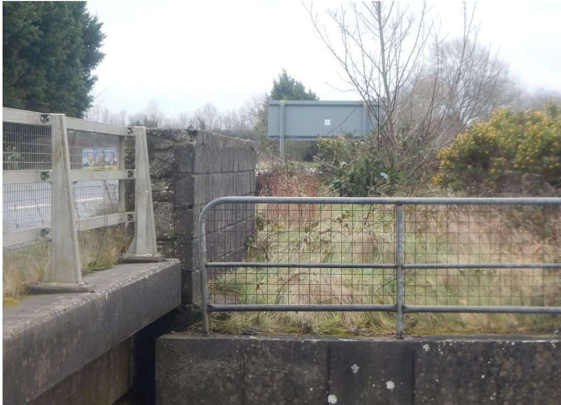
Photo 31 – Structure 2: Masonry Parapet Wall at Southeast Corner
