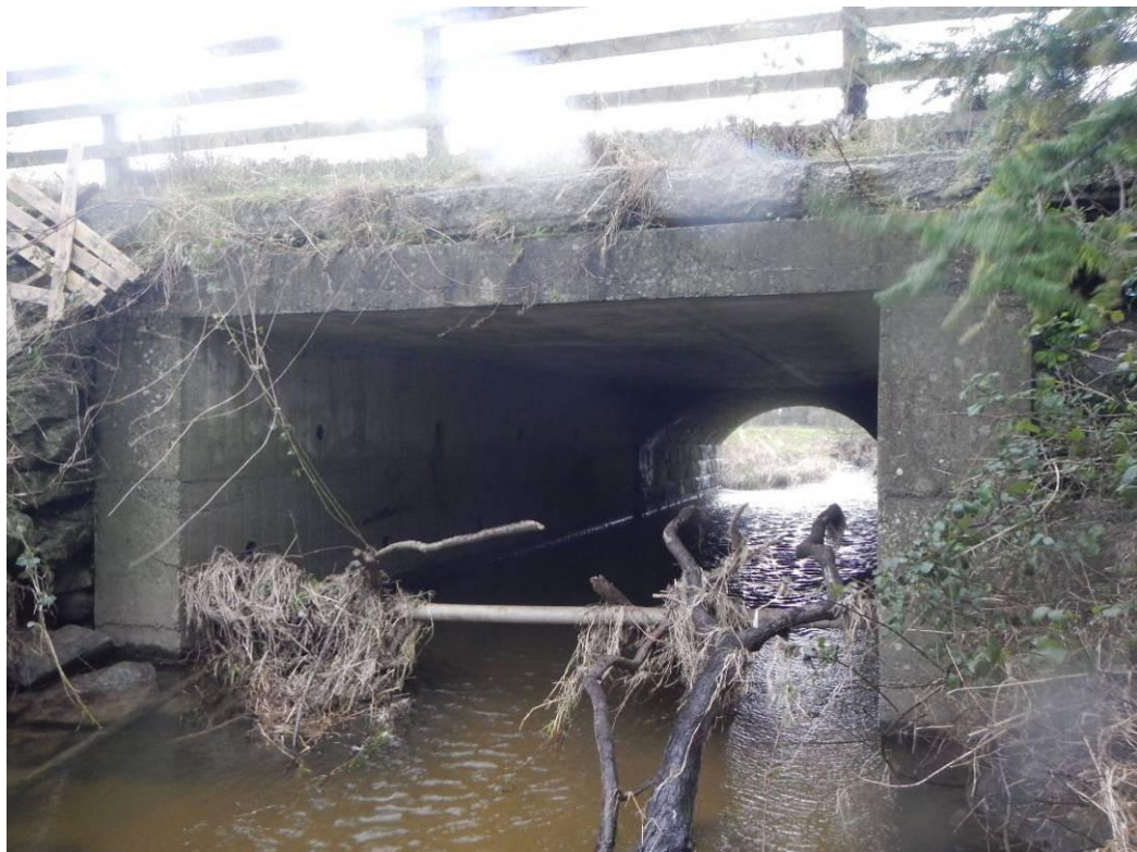
Photo 14 – Structure 1: East Elevation
