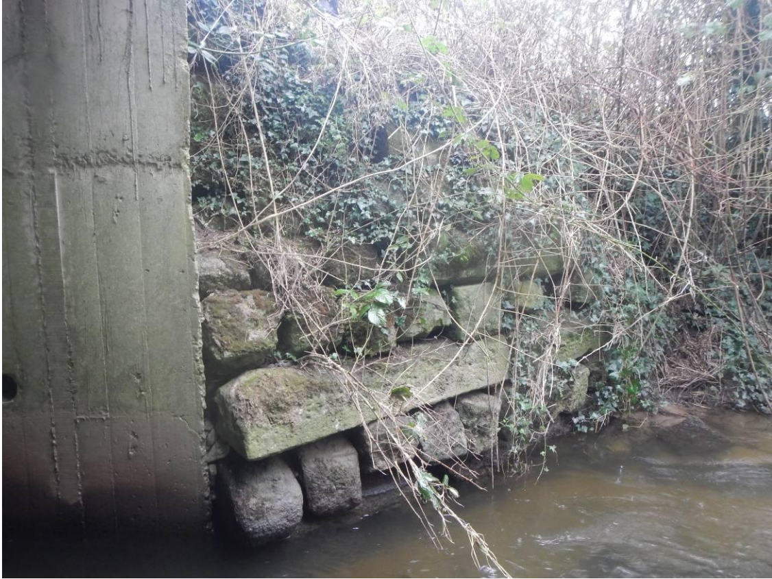
Photo 37 – Structure 3: Southwest Masonry River Training Wall
