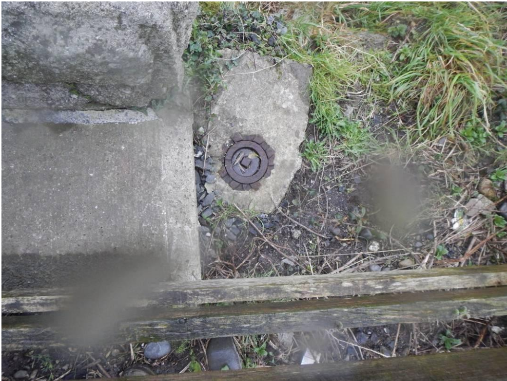
Photo 4 – Structure 1: View of Scour Valve in West Verge
