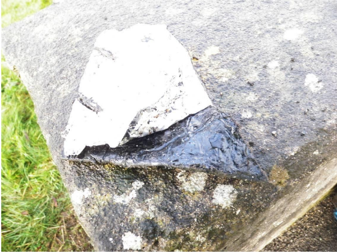
Photo 29 – Structure 2: Waterproofing From Structural Investigation
