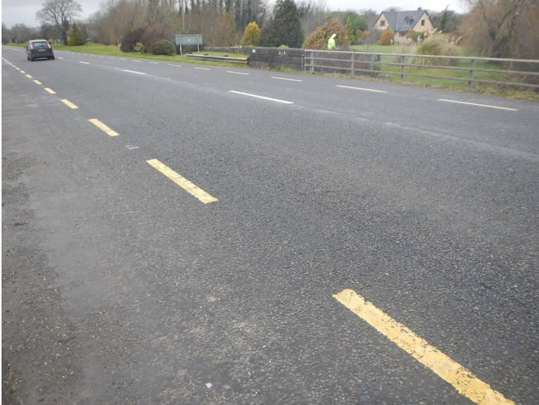
Photo 17 – Structure 2: View of Carriageway Surfacing
