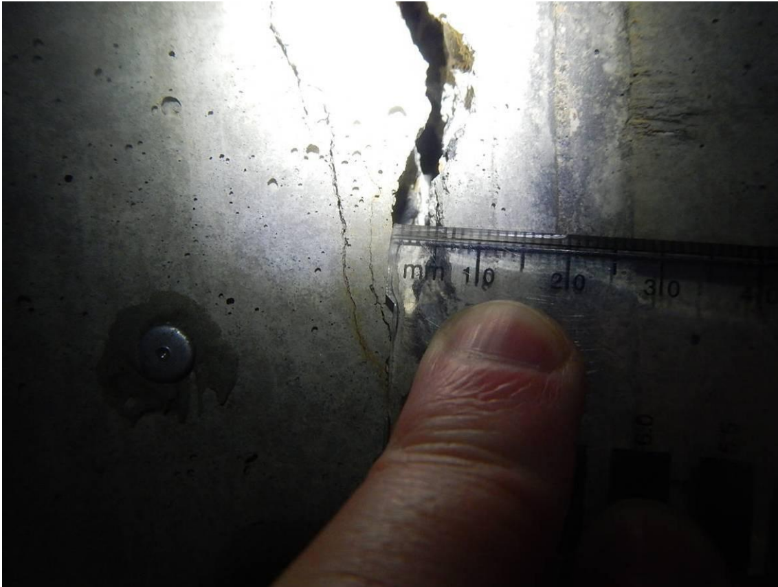
Photo 66 – Structure 4: Cracking on Abutment
