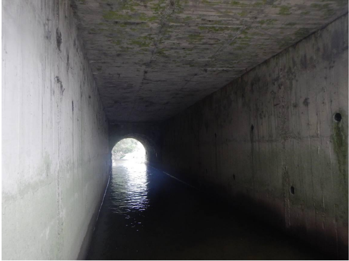
Photo 43 – Structure 3: View on Concrete Abutments
