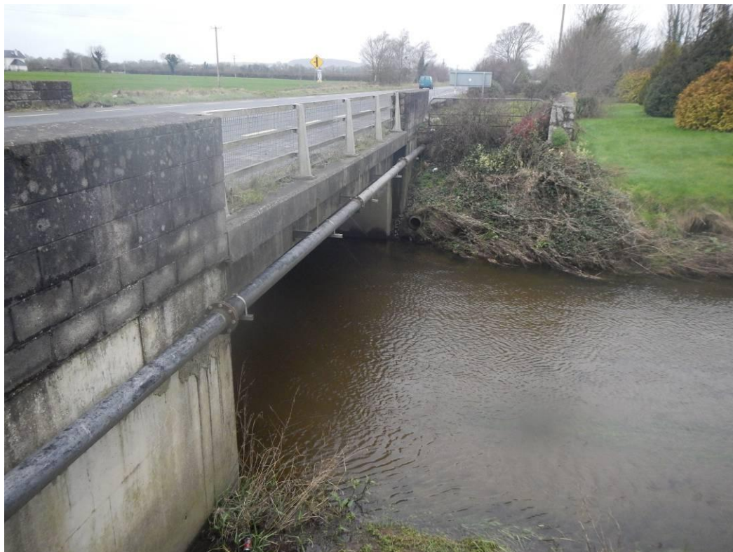
Photo 20 – Structure 2: Watermain on North Face
