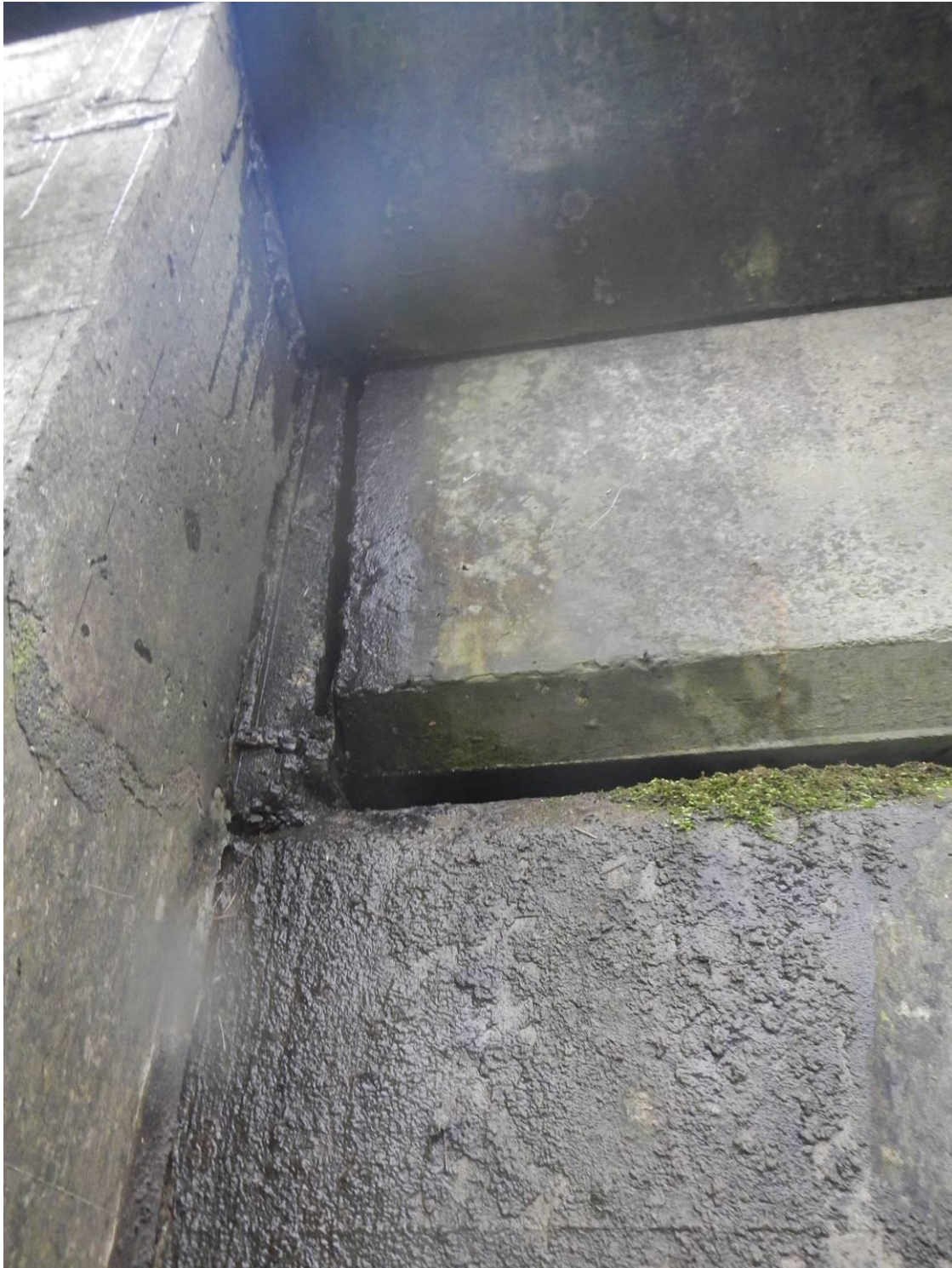
Photo 26 – Structure 2: Leakage Above Abutment at Northeast Corner
