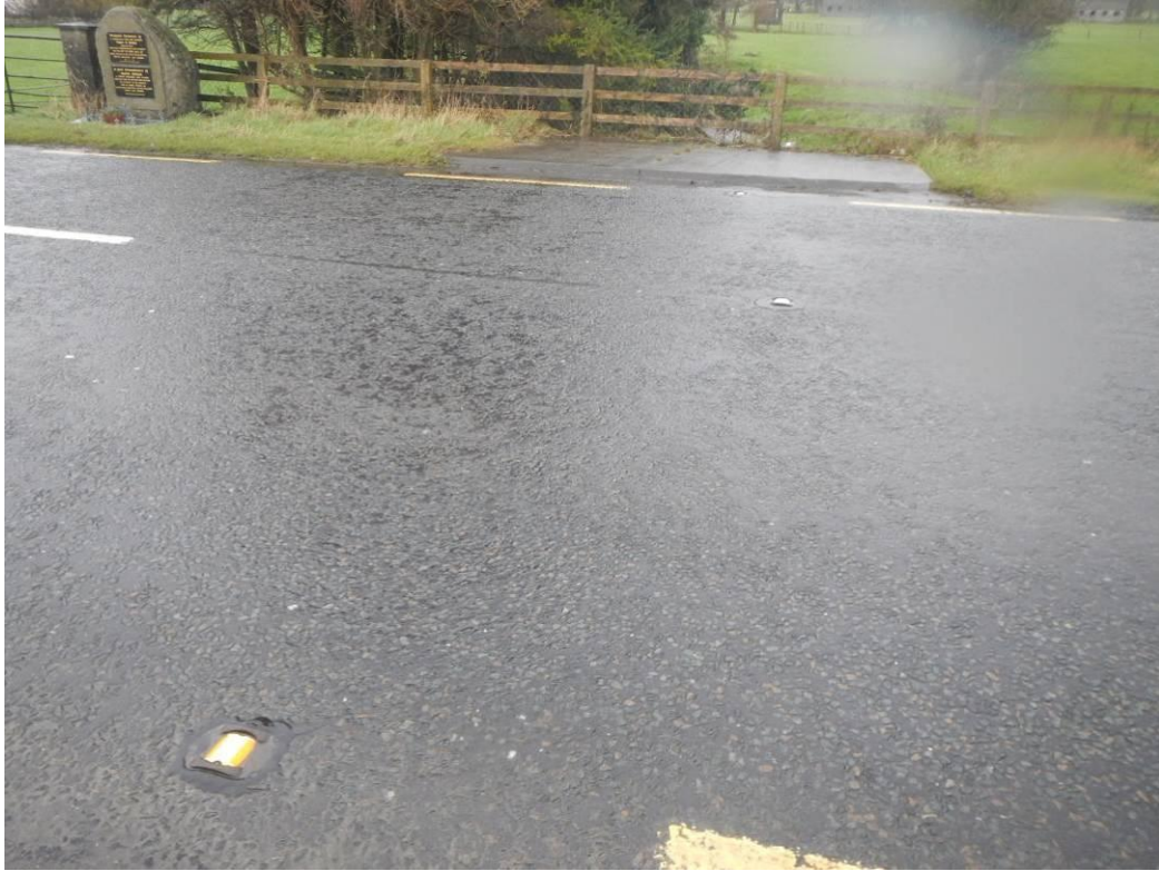
Photo 1 – Structure 1: View of Carriageway Surfacing
