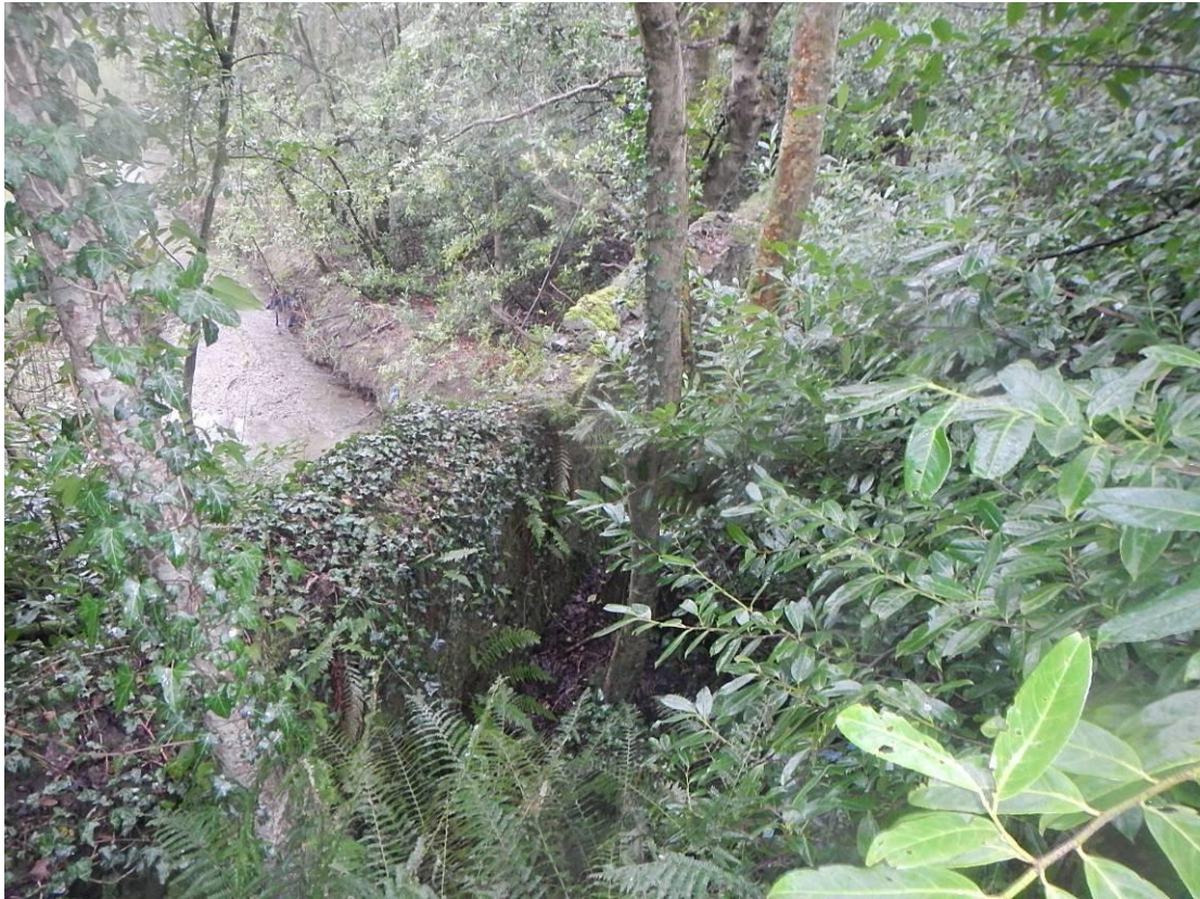
Photo 49 – Structure 4: View on West Masonry Parapet
