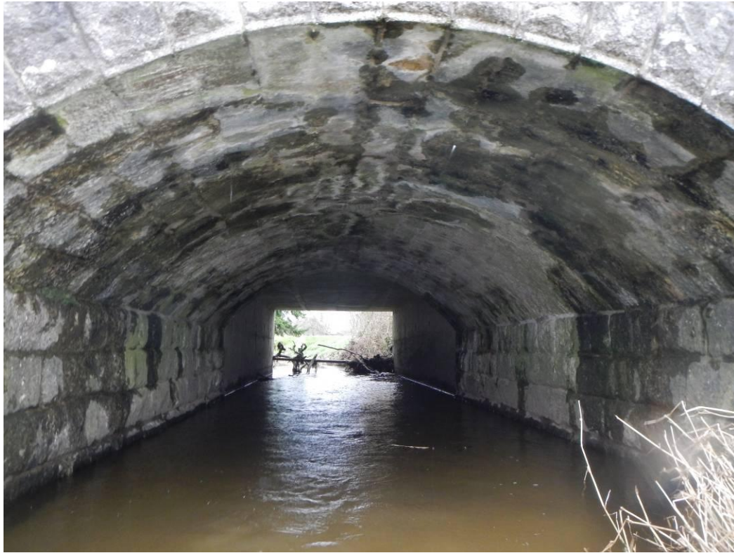
Photo 9 – Structure 1: View of Arch Barrel facing East
