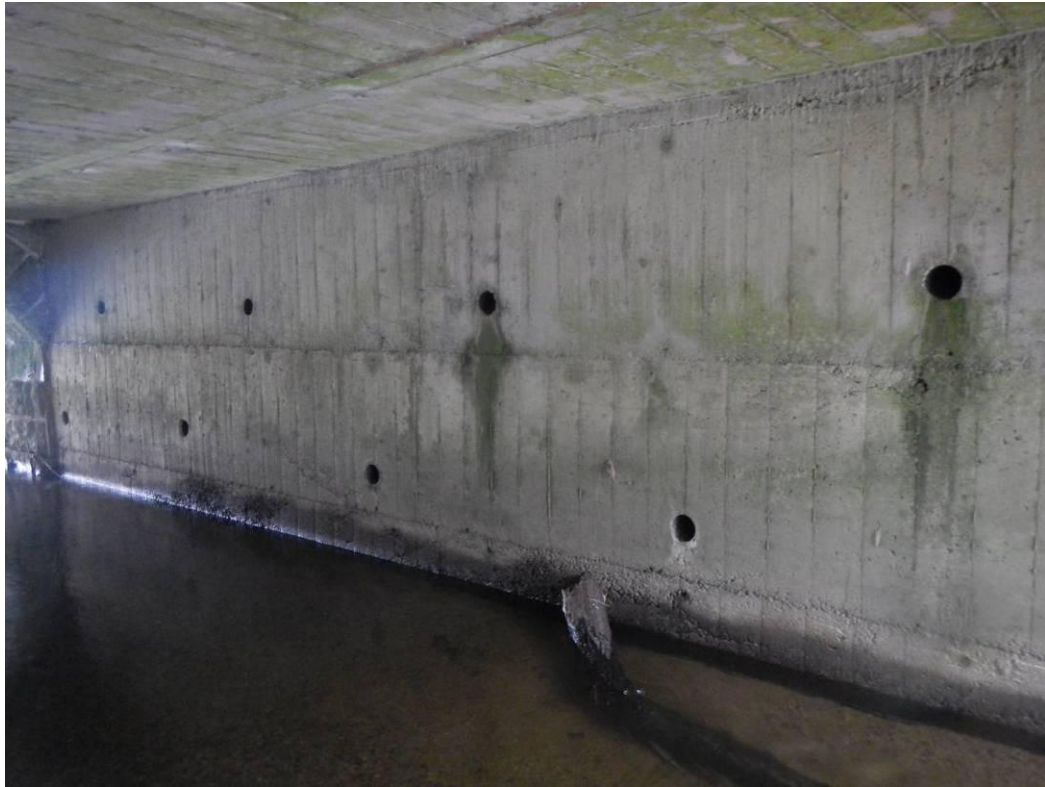
Photo 13 – Structure 1: Concrete Abutment
