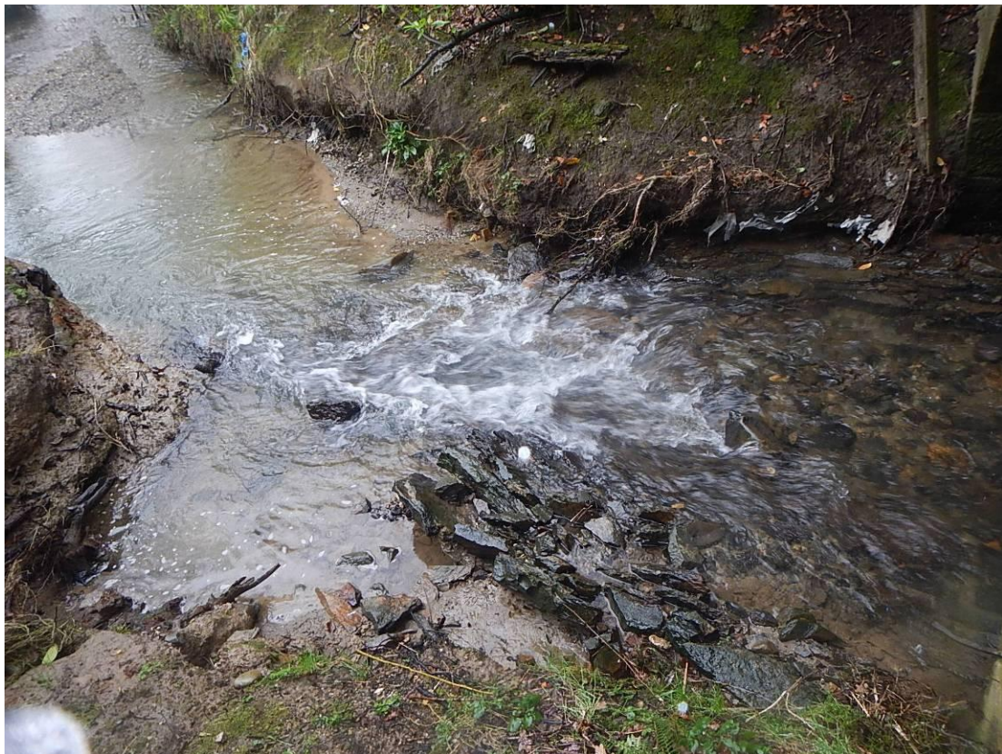
Photo 67 – Structure 4: View on Downstream
