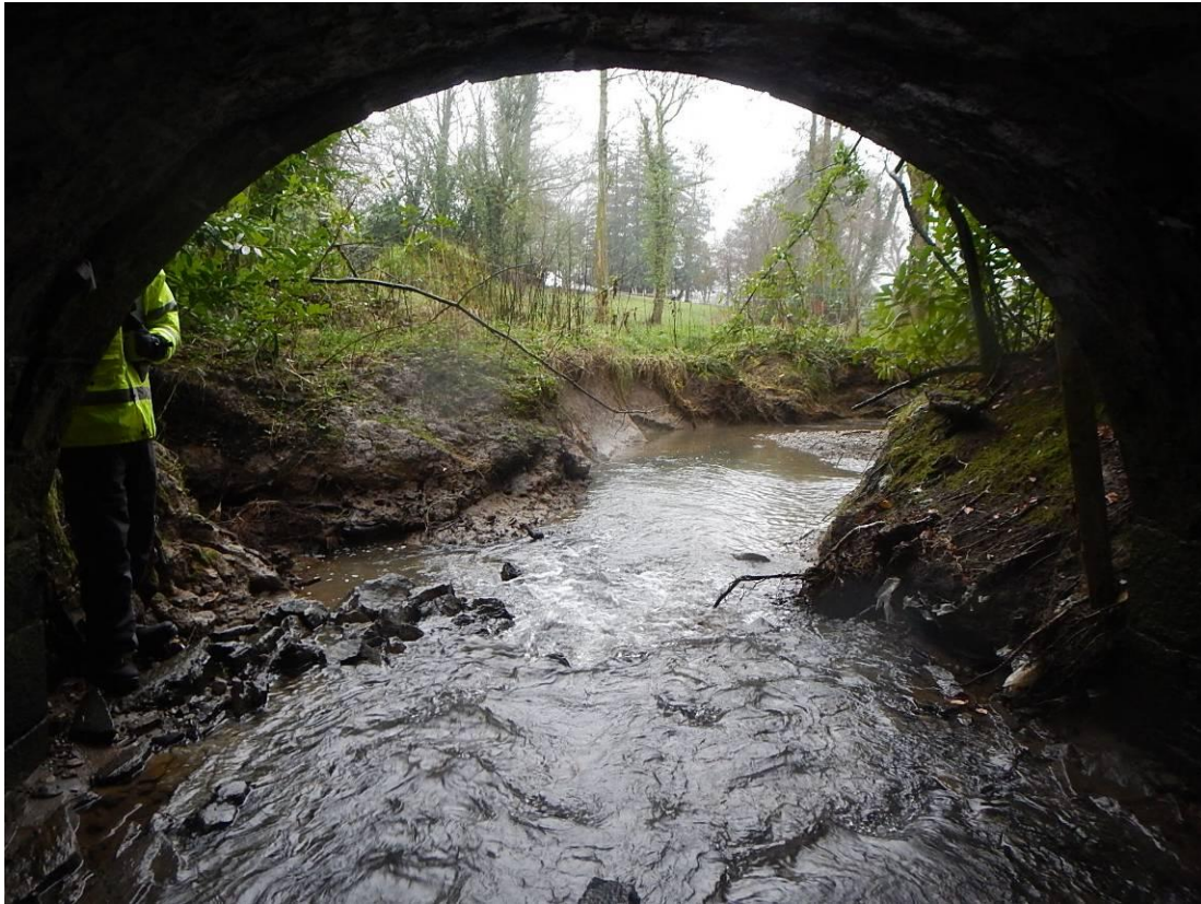
Photo 53 – Structure 4: Erosion of Southwest Embankment
