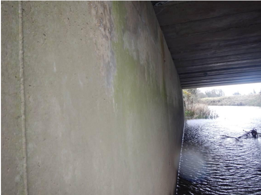
Photo 27 – Structure 2: Staining on East Abutment
