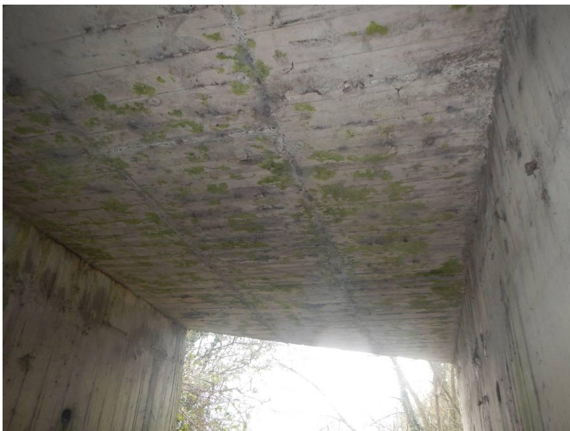
Photo 40 – Structure 3: Reinforced Concrete Deck
