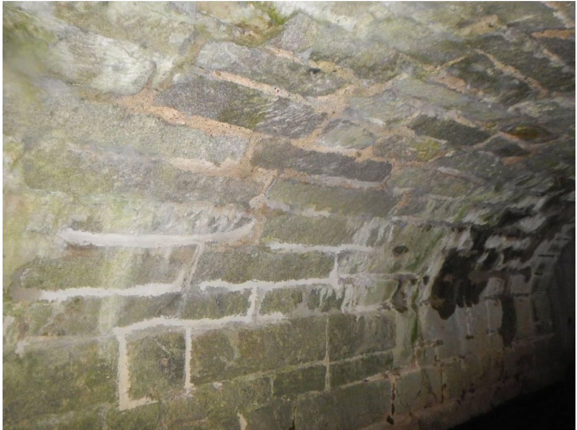
Photo 42 – Structure 3: Southern Masonry Abutment
