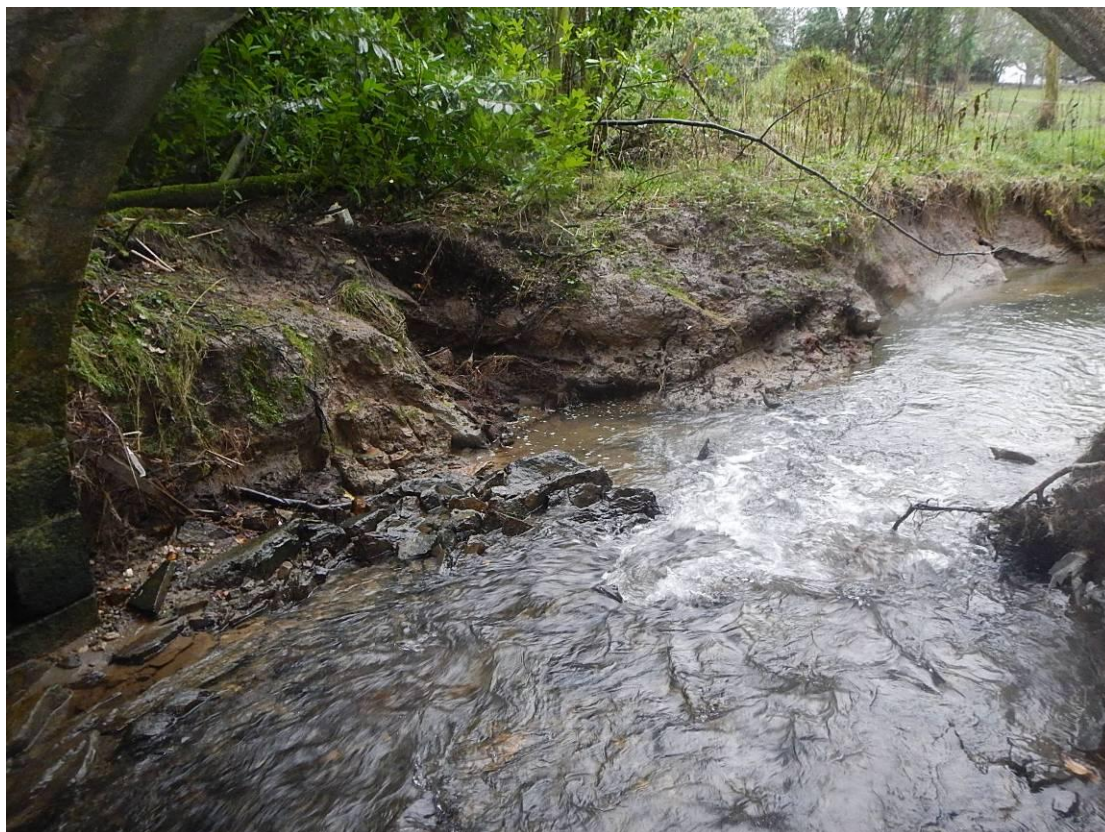
Photo 68 – Structure 4: View on Downstream
