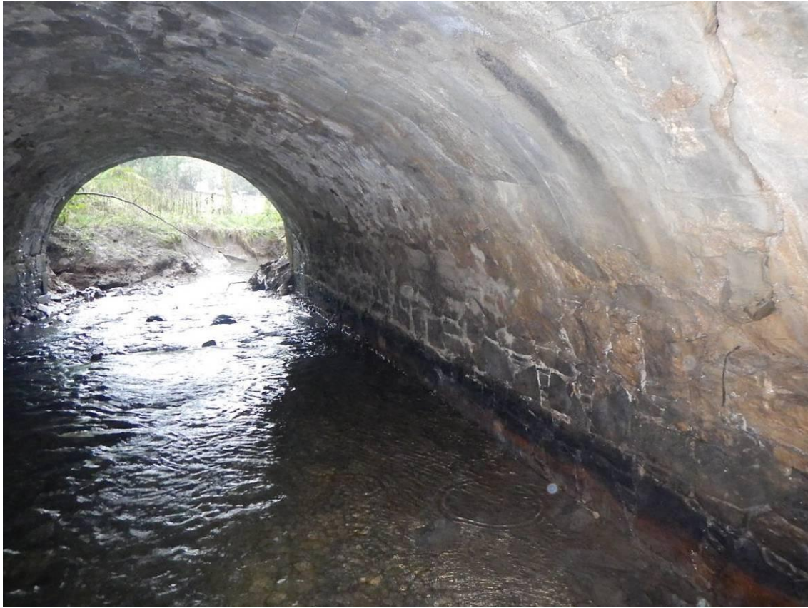
Photo 62 – Structure 4: Masonry Abutment
