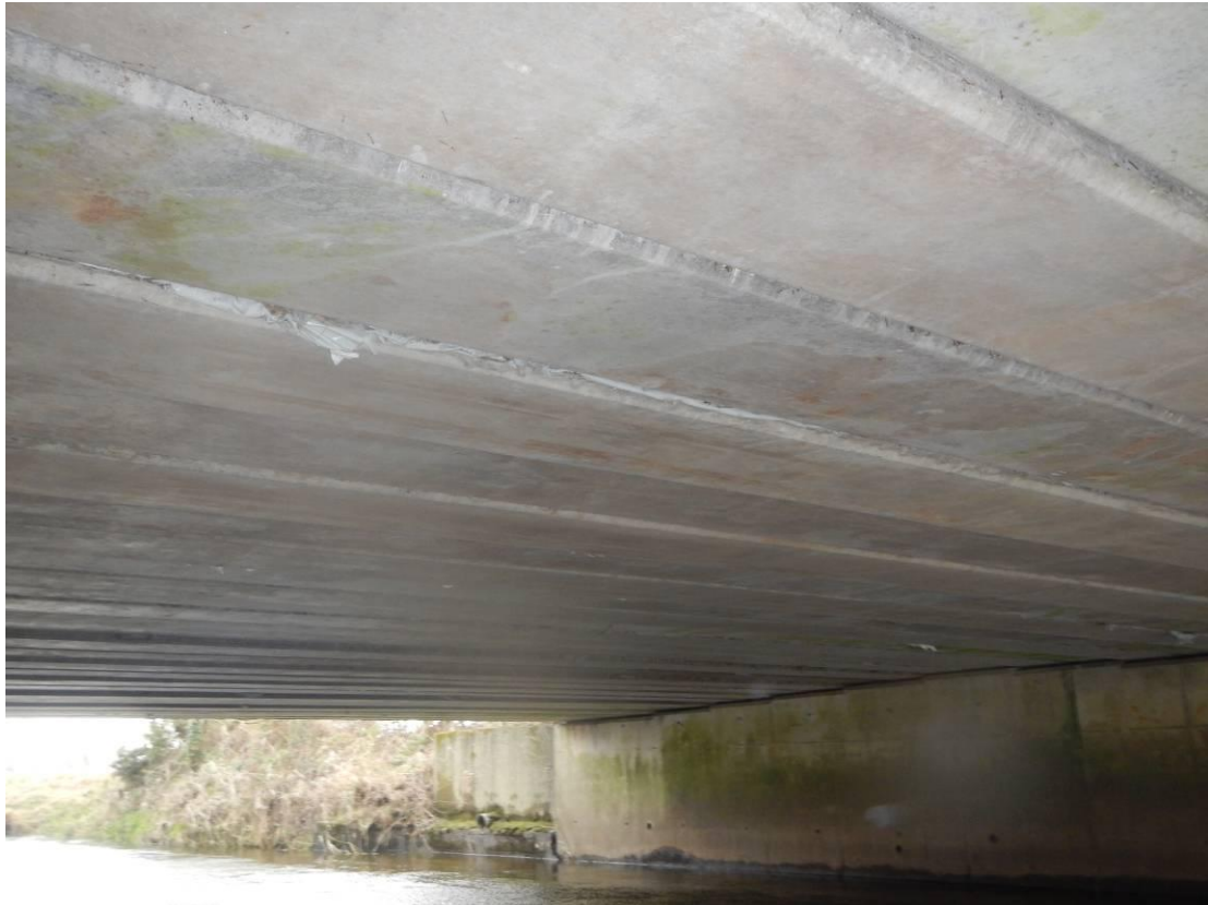
Photo 23 – Structure 2: Bridge Soffit
