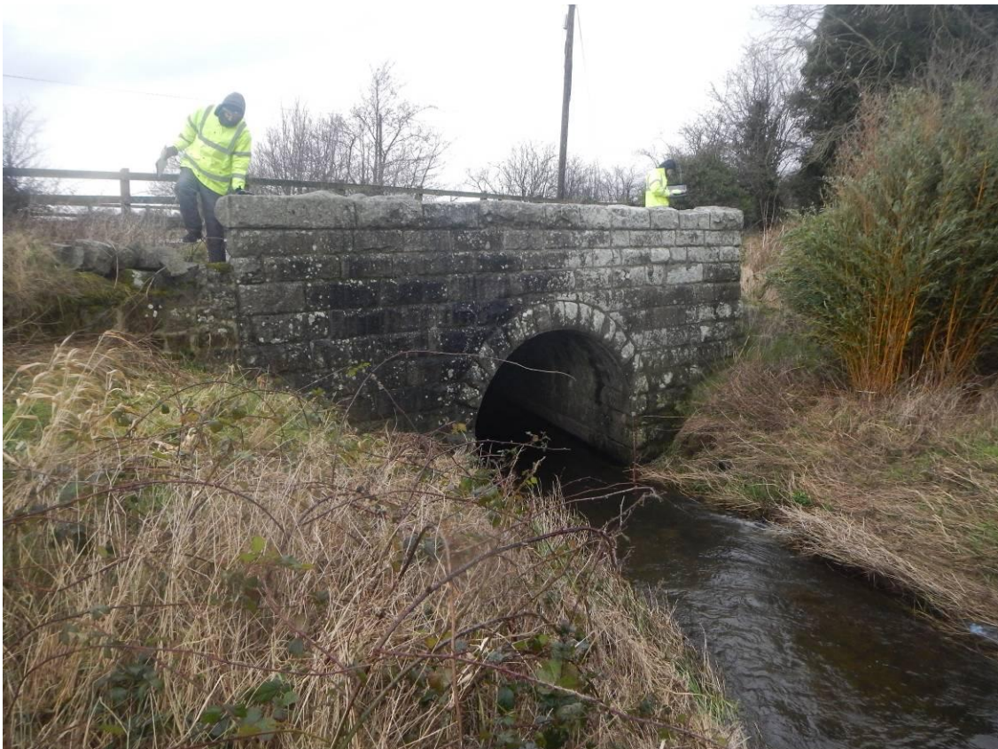
Photo 44 – Structure 3: East Elevation
