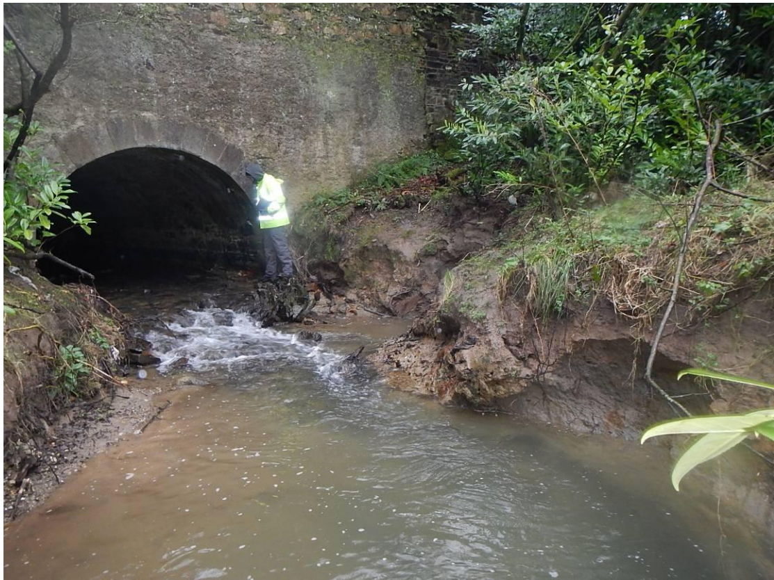
Photo 52 – Structure 4: Erosion of Southwest Embankment
