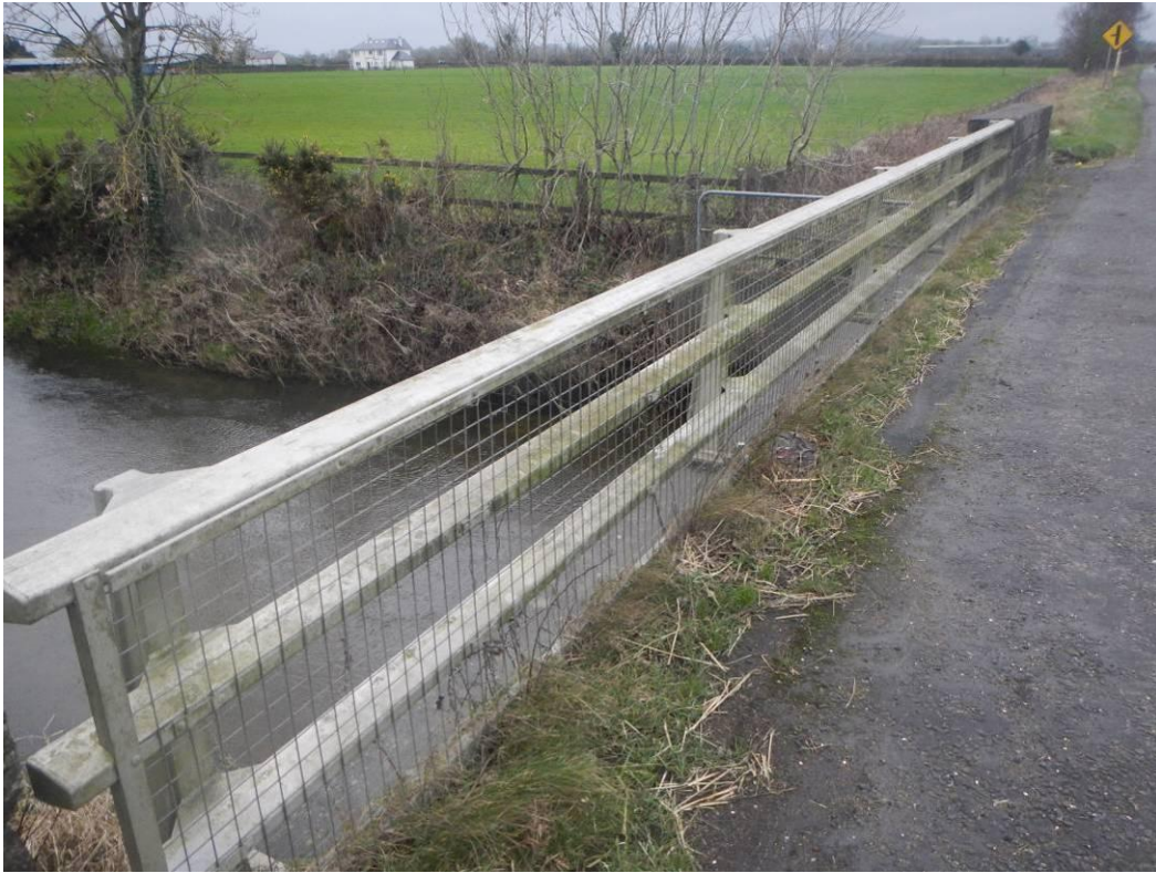
Photo 19 – Structure 2: View of South Parapet
