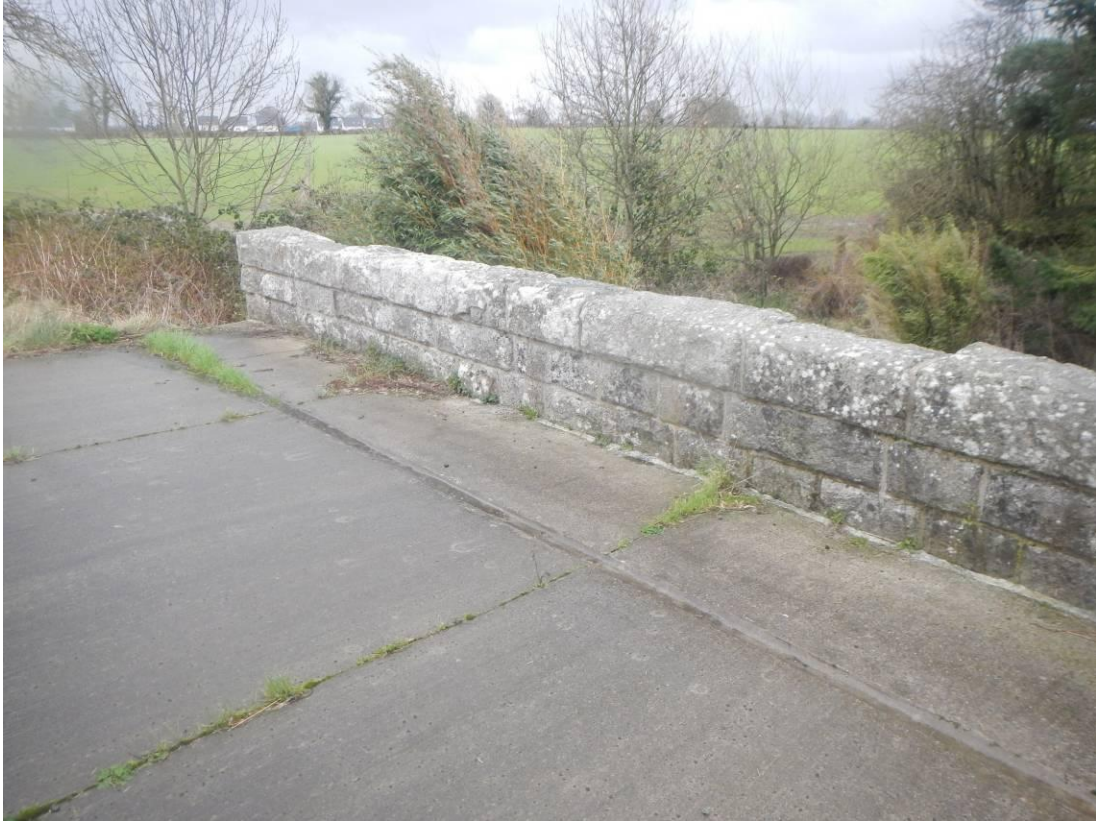
Photo 33 – Structure 3: Eastern Masonry Parapet Wall
